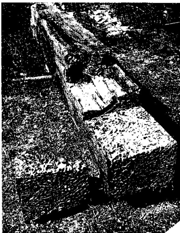
FIG. 10. — Marine borer damage to Panama Canal fender timbers, Miraflores Locks, untreated pine.
