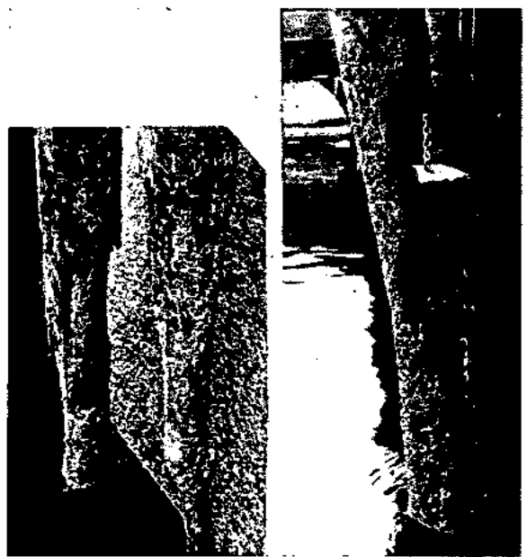
FIG. 1. — Examples of marine borer damage to wooden structures in Canal Zone waters. Creosoted piling, Balboa Harbor of the Pacific entrance of Panama Canal, low tide view.
