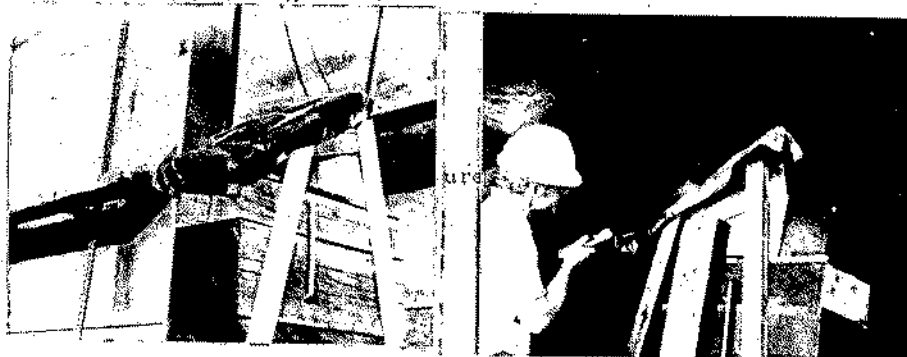
Figure 10 - Typical Dok-Blok Tape System on the Side Block of the Ferry Boat, Before and After Dry Docking
